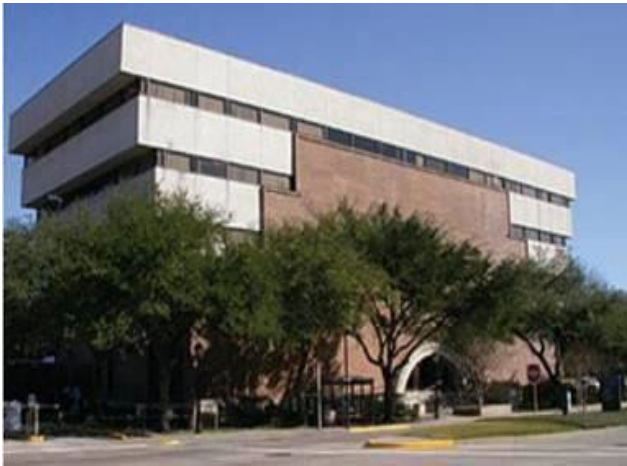
University of Houston TMC Renovation Project
