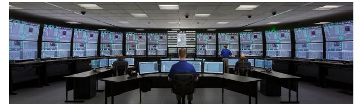
NuScale Control Room Simulator
