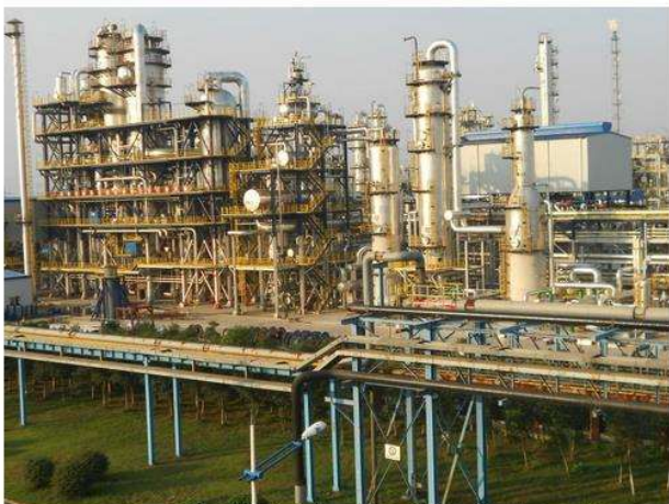
Honeywell UOP started its first MTO unit for China's Wison Clean Energy in 2013 photo credit: Honeywell UOP
